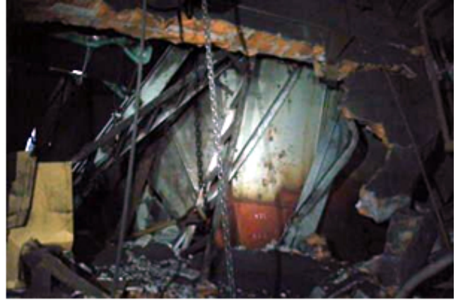
Damage sustained at Fukushima Steel Work Co., Ltd.
