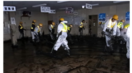
Cleaning mud inside an office
