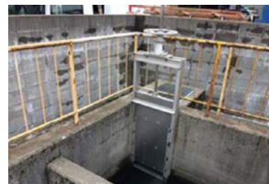
Blockade dam for preventing abnormal drainage
