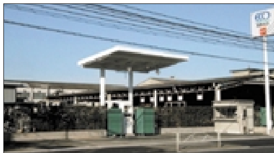
■ Hino Motors Eco-Station Supply capacity: 250 Nm 3 /h (For about 50 units of light-duty truck or 40 units of medium-duty truck per day)
