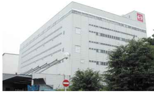
Oume Parts Center Maintains replacement parts for trucks and buses, shipped all over the country.
