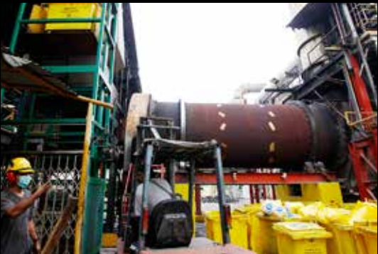
Incinerator for processing medical waste. Medical waste is incinerated shortly after being transported here, and what cannot be quickly incinerated is stored in a refrigerated warehouse.
