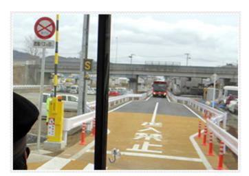
The designated BRT driving lane can be seen from the driver's seat. Gates were built to prevent other vehicles from mistakenly entering the designated road
