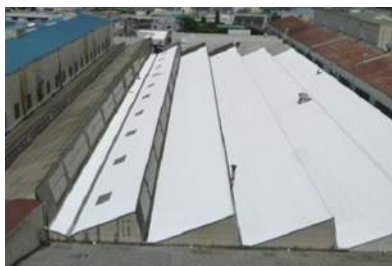
Roof with thermal barrier coating
