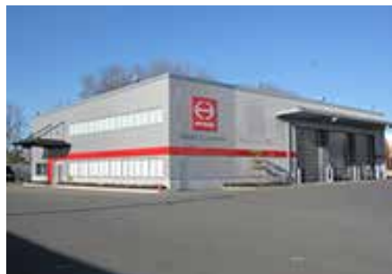
The Customer Technical Center
