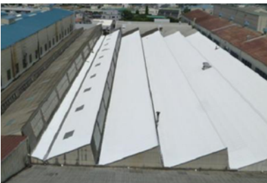
Roof with thermal barrier coating
