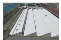
Roof with thermal barrier coating
