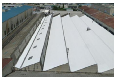
Roof with thermal barrier coating
