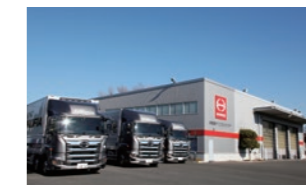
The Customer Technical Center
