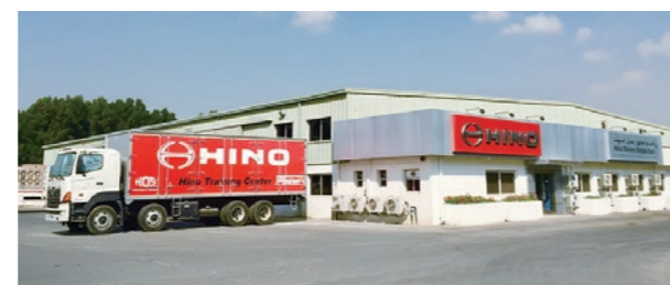
Hino Training Center – Middle East
