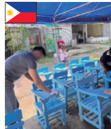
Repairing chairs in an elementary school (Hino Motors Philippines Corporation)
