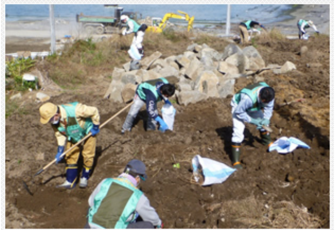
Work in process
