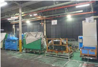
Soundproof sheets installed in the plant building
