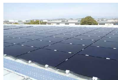
The roof of the new cafeteria
