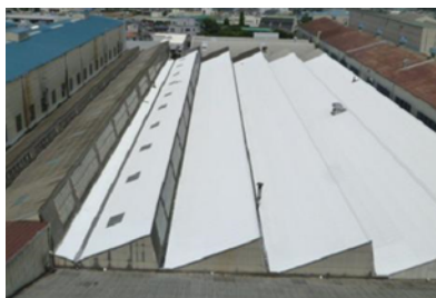
Roof with thermal barrier coating
