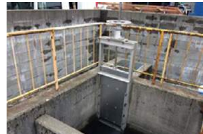
Blockade dam for preventing abnormal drainage
