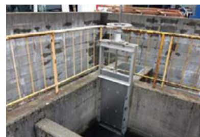
Blockade dam for preventing abnormal drainage
